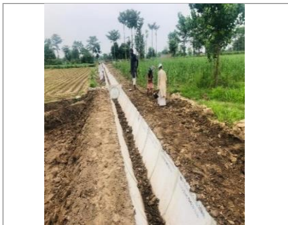
Figure 4.53: Proper back filling of watercourse 11430/R
