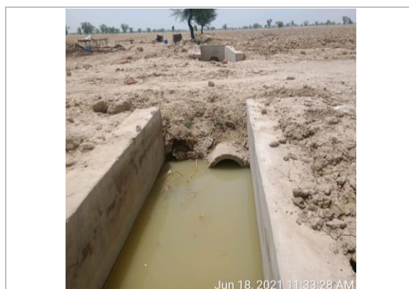
Figure 4.91: Concrete Culvert with Watercourse
