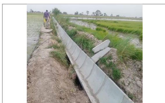
Figure 4.59: Slope issue at Watercourse in Kalianwala of watercourse no18715/R
