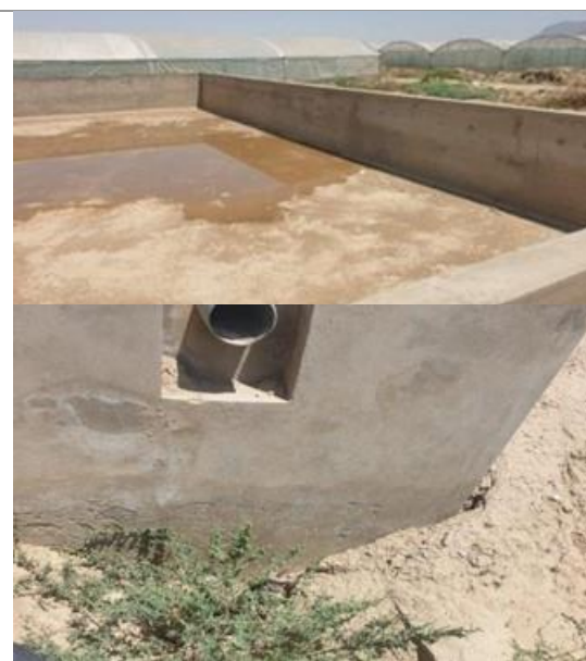
Picture 3.69: View of WST showing pile of mud inside outflow and was not in use at all.
