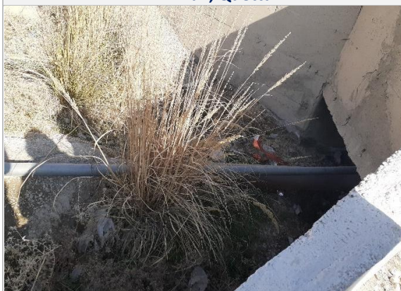
Figure-5.29: View of pipe passing through under Bypass Road
