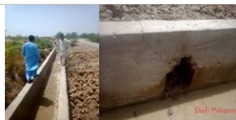
Picture 4.107: View of Watercourse with Damaged Portion, Sohbatpur, Balochistan
