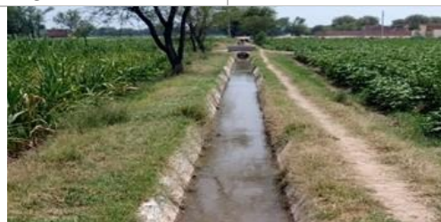
Picture 4.22: Improper Cleaning of W/C 106200 L
