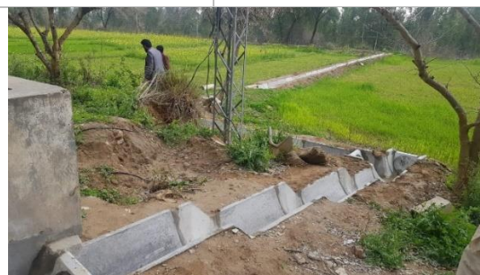
Picture 4.15: Channi Kanjal Watercourse Under Construction
