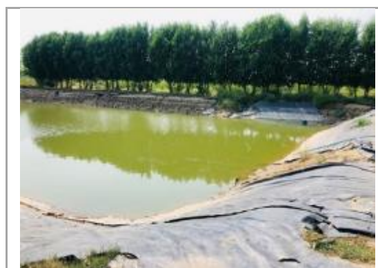
Figure 3.12: Eroded View of Geomembrane WST
