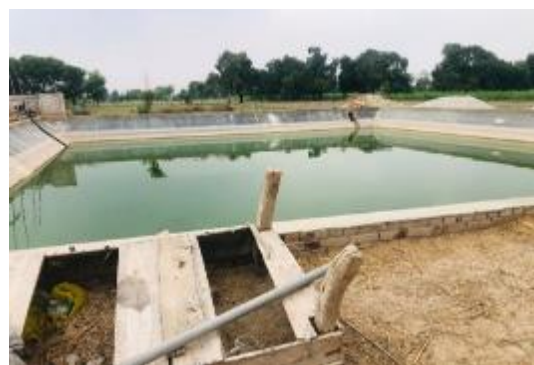
Pictorial View of Concreted WST
