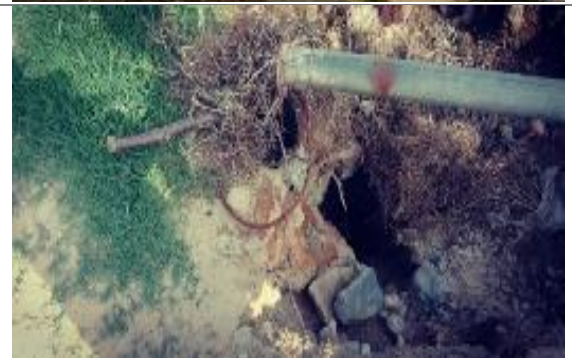
View of damaged PVC Pipes, District Loralai
