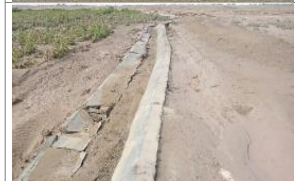
View of damaged PVC Pipe and Watercourse, District Kharan
