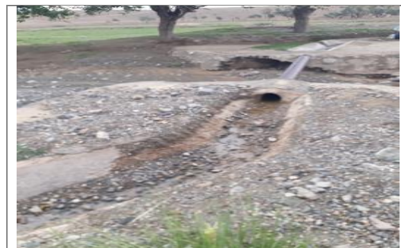
View of damaged PVC Pipe and Watercourse, District Kharan
