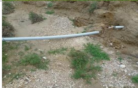
View of damaged PVC Pipe, District Mastung
