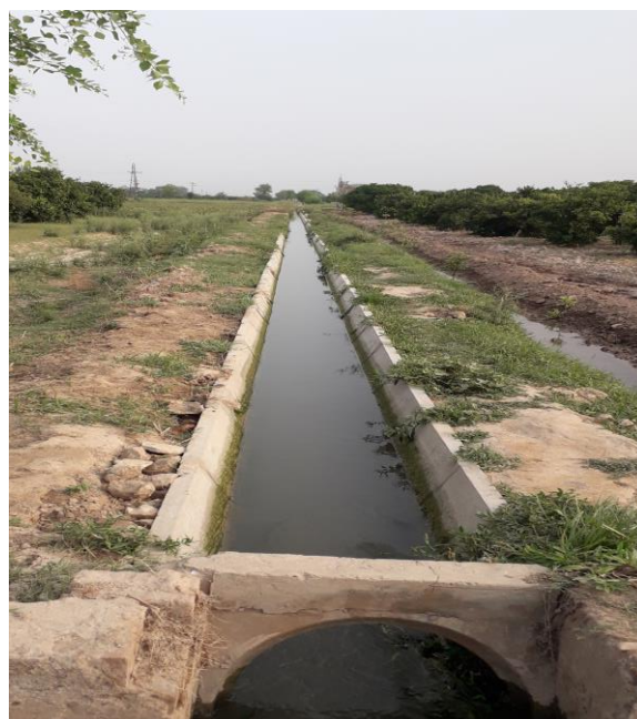
28240/L View of Proper Earth filling of Sides of Watercourse
