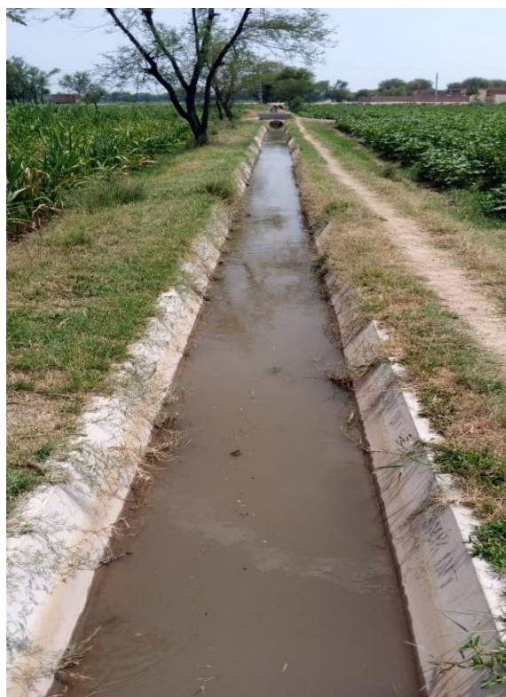
Improper Cleaning of W/C 106200 L
