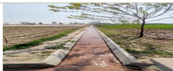
A view of the lined portion of the Watercourse
