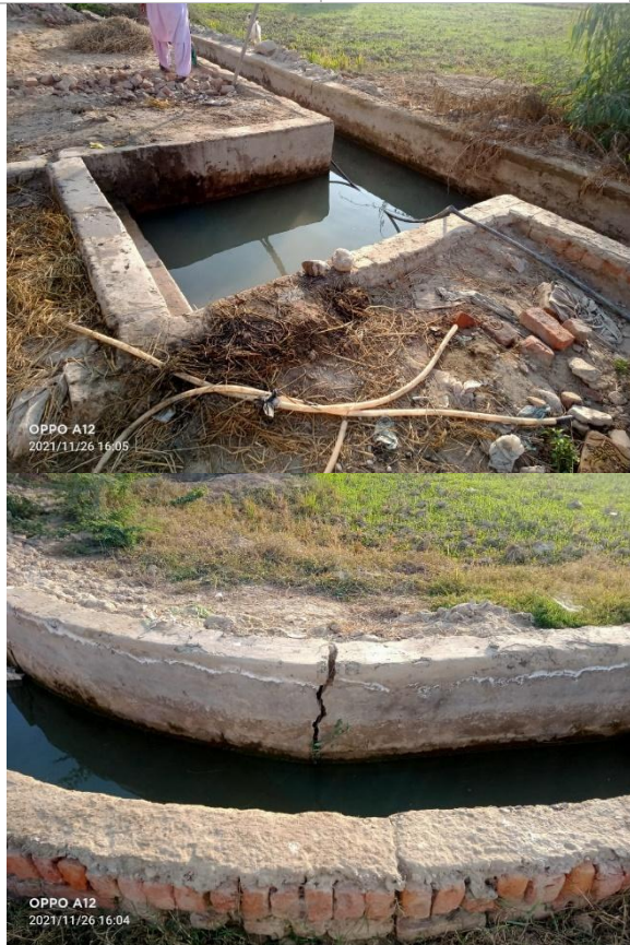
View of cracks in Watercourse and measuring length of WC
