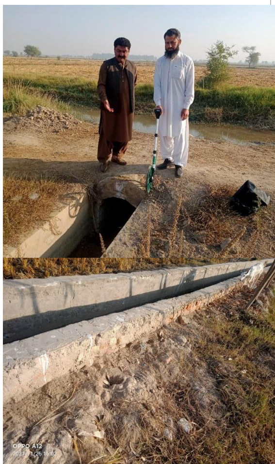
Measuring the WC and view of backfilling not done properly and bad quality of plaster
