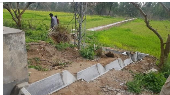
Figure 4.19: Channi Kanjal Watercourse Under Construction
