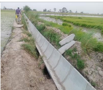
Figure-4.59: Slope issue at Watercourse In Kalianwala of watercourse no18715/R
