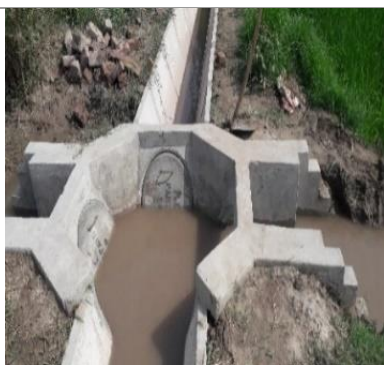
Figure-4.41: Improper back filling of watercourse 3854/L Kasur
