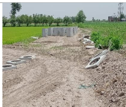
Figure-4.56: Improper placement of Segments & Naccas on watercourse no 21600-R
