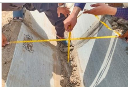
Figure-4.74: Checking depth of WC 63100/L
