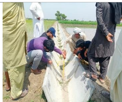
Figure-4.63: Checking the depth of Watercourse no 12445/R Dellah Chatha
