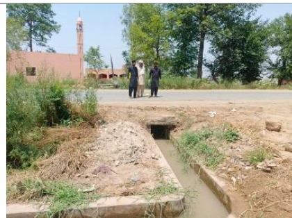
Figure-4.64: Culvert is provided under the road of Watercourse no 12445/R
