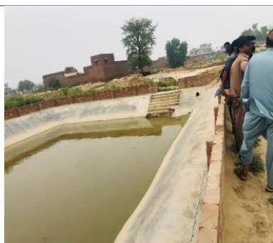
Figure-4.43: View of Concreted WST
