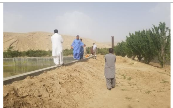
Figure-4.153: View backfilling of WST
