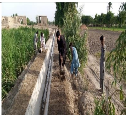
Figure-4.84: Backfilling process in progress at water course 94934 L
