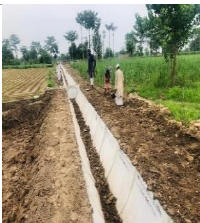
Figure-4.51: Proper back filling of watercourse 11430/R
