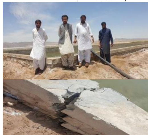
Spot checking of WST with OFWM staff. Boundary of WST is damaged
