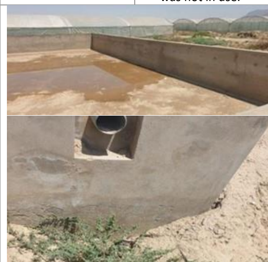
View of WST showing pile of mud inside outflow and was not in use at all.
