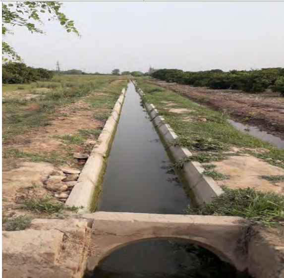
Figure 4.11: 28240/L Proper filling Water course sides
