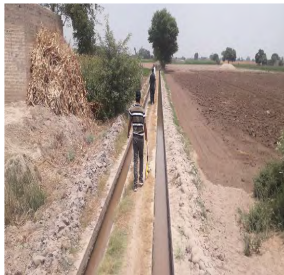
Figure 4.14: Measuring Lining Length of Water Course with Measuring Wheel
