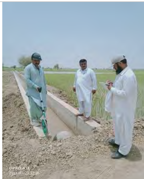
Figure 4.34: Measuring Watercourse
