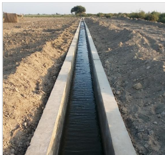
Figure-7.2: View of a constructed lined watercourse
