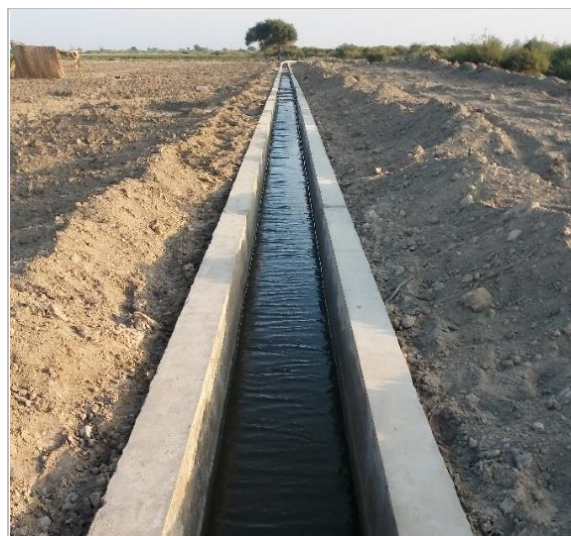
Figure-7.2: View of a constructed lined watercourse
