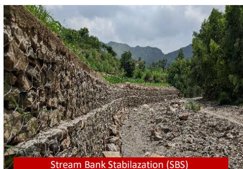
Stream Bank Stabilization (SBS)
