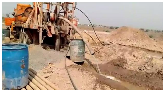
Figure-5.1: Development of Tube Well for Mr. Gul Said Tube Well & Solarization of Tube Well in Maraje Mankisharif, Nowshera
